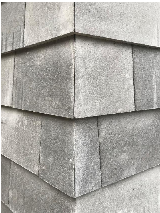
Picture of example 4, corner without aluminium flashing
